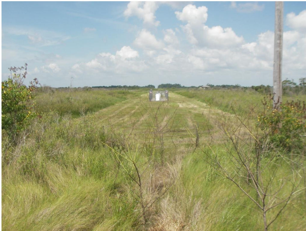
East Pumping Facility
