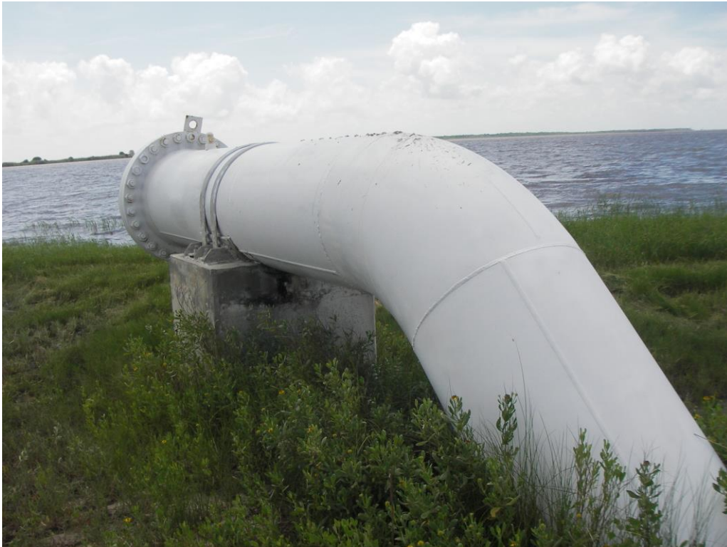
East End Blind Flange/Riser Pipe
