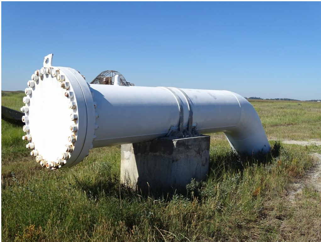
East End Blind Flange/Riser Pipe
